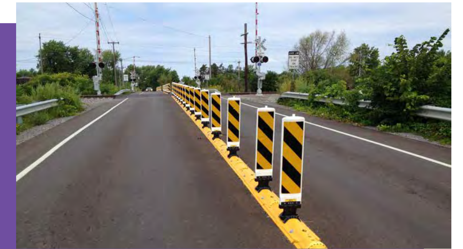
Example: Quiet Zone Crossing Delineators and Quad Gates
